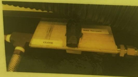
House Vacuum Valve and Gauge
