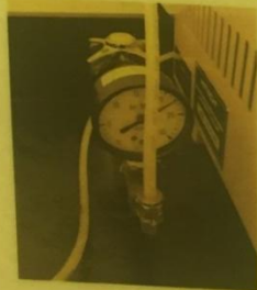
House Vacuum Valve and Gauge
